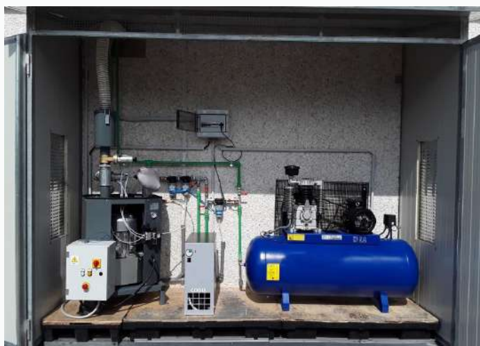
Soffiante a canale laterale in locale tecnico Separated side channel blower unit in technical environment
